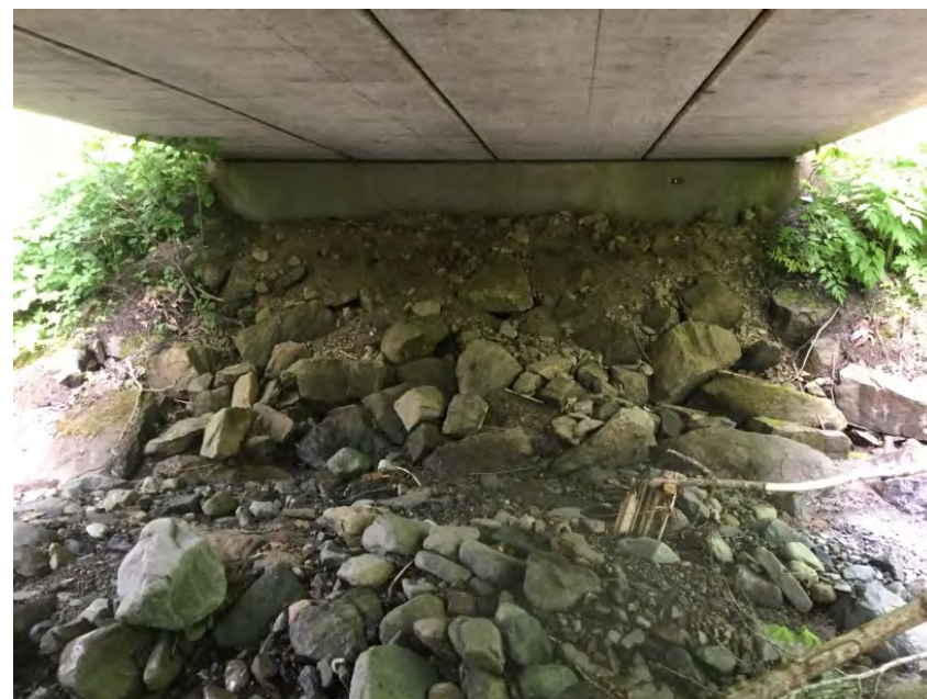
Right Bank Abutment when facing downstream
