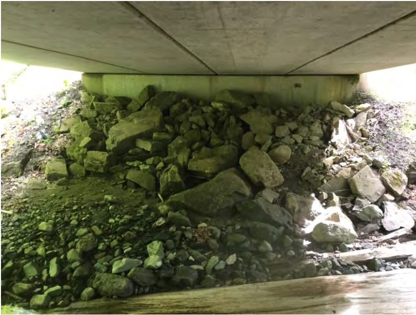
Left Bank Abutment when facing downstream
