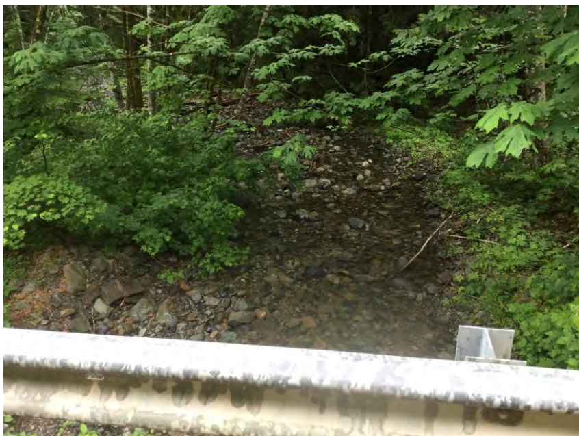
Looking downstream from deck
