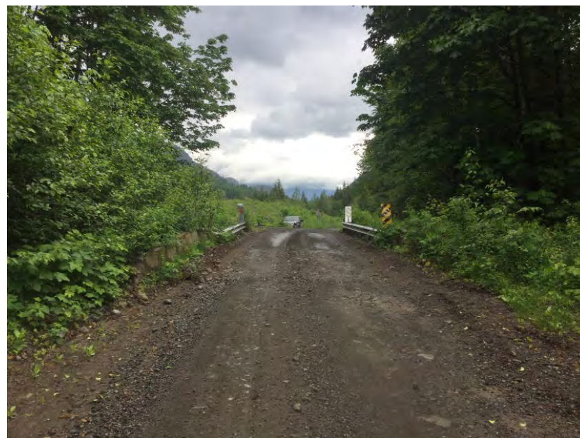
Approach from Right Bank when facing downstream
